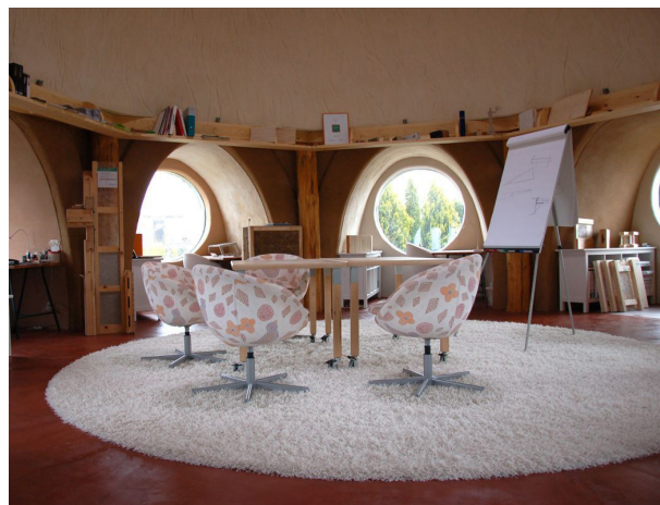
Figure 4.3.10 Self-bearing Straw bale dome made in passive standard, in Hrubý Šúr, Slovakia, is the headquarter of the architecture studio Createrra, made of natural renewable materials: straw bales as the main construction material, wood structure, with using of green roof on the top, clay floor finished with flax oil varnish, walls covered by clay plaster (Createrra)
