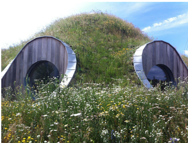
Figure 4.3.10 Self-bearing Straw bale dome made in passive standard, in Hrubý Šúr, Slovakia, is the headquarter of the architecture studio Createrra, made of natural renewable materials: straw bales as the main construction material, wood structure, with using of green roof on the top, clay floor finished with flax oil varnish, walls covered by clay plaster (Createrra)
