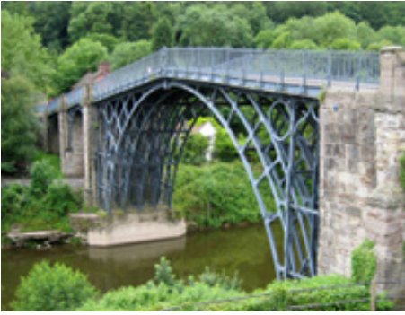
Figure 5.1.6 First metal bridge over River Seven
