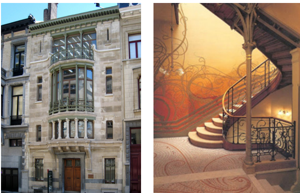
Figure 5.1.12 Exterior and interior views of Hôtel Tassel
