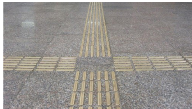
Figure 3.3.9 a, b Artificial guiding lines – metal tactile indicators (Dessau, Germany and Poprad, Slovakia, Čerešňová)
