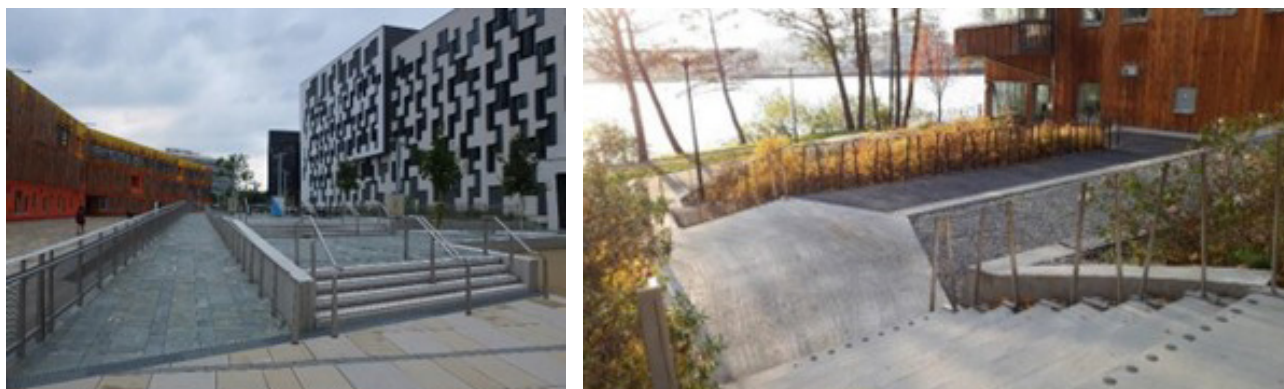
Figure 3.3.12 a, b Ramps situated next to the stairs (Vienna and Stockholm, Čerešňová)
