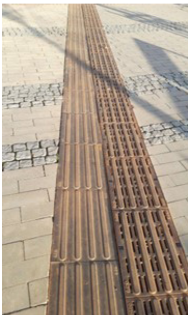
Figure 3.3.10 a, b Artificial guiding lines – tactile tiles with drainage (Stockholm and Copenhagen)
