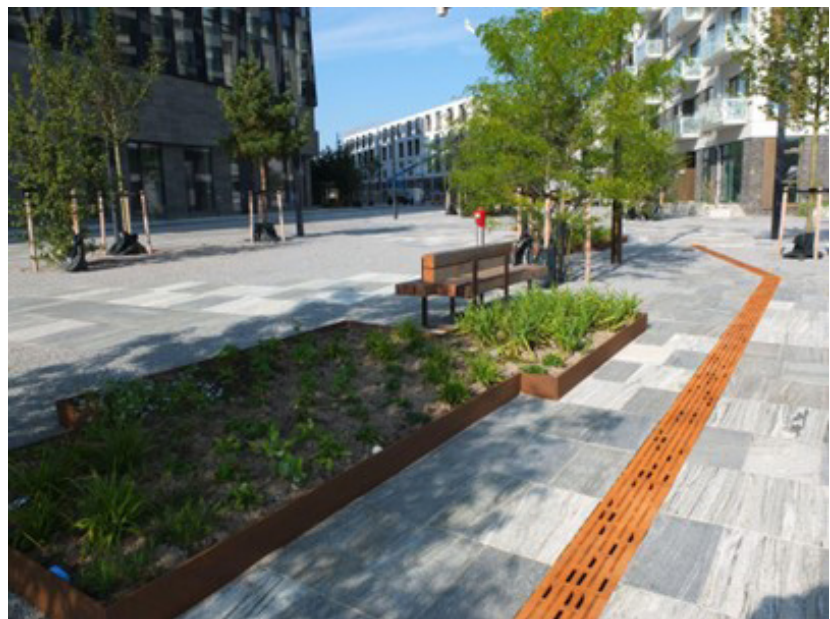
Figure 3.3.10 a, b Artificial guiding lines – tactile tiles with drainage (Stockholm and Copenhagen)
